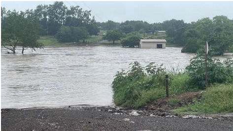
Figure 3: A flooded pump house on one of our members' farms.
